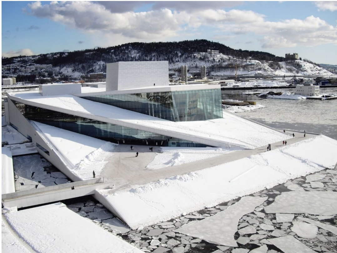
Figure 4.27. Oslo Opera House, Snøhetta, Oslo, 2000-2008.
